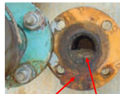
Sand build up in pipework
