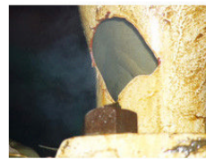
Choke Damage Internal
